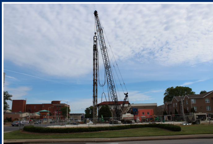
In July, ninety six 50+ footers were poured as part of the foundation for the 3-story C.E. Field Center.
